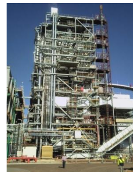
Main boiler building
