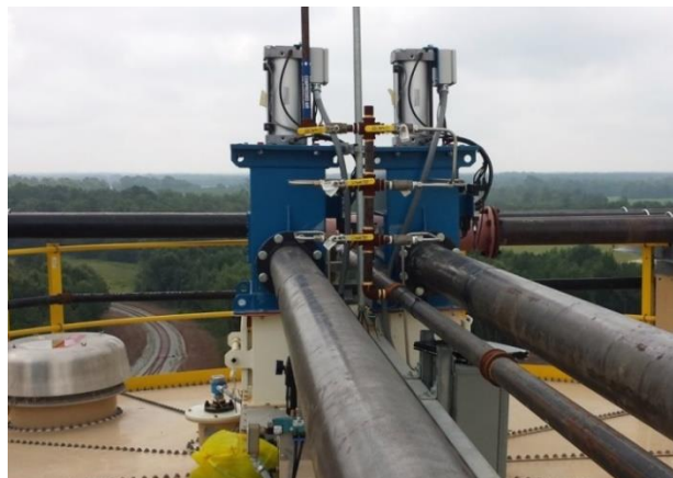
Diverter valves on the reception silo
