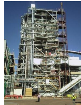
Main boiler building
